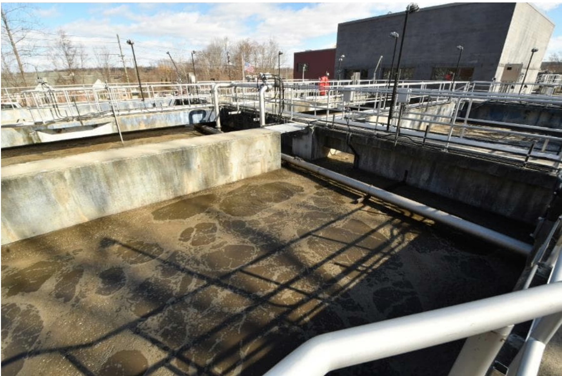
Aeration Tank No. 1 with Blower Building Maintenance Garage Behind
