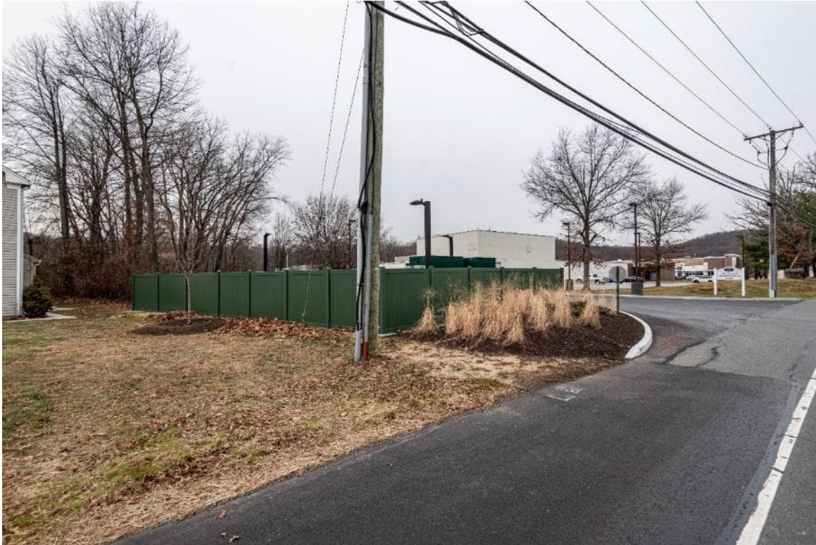
Pump Station Looking Northwest
