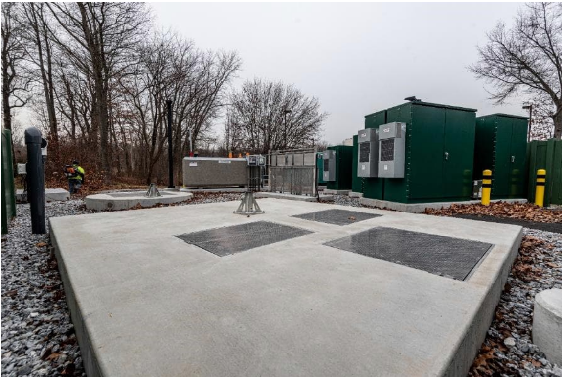
Pump Station Site
