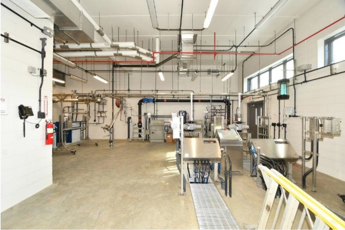
UV Disinfection / Reaeration Building
