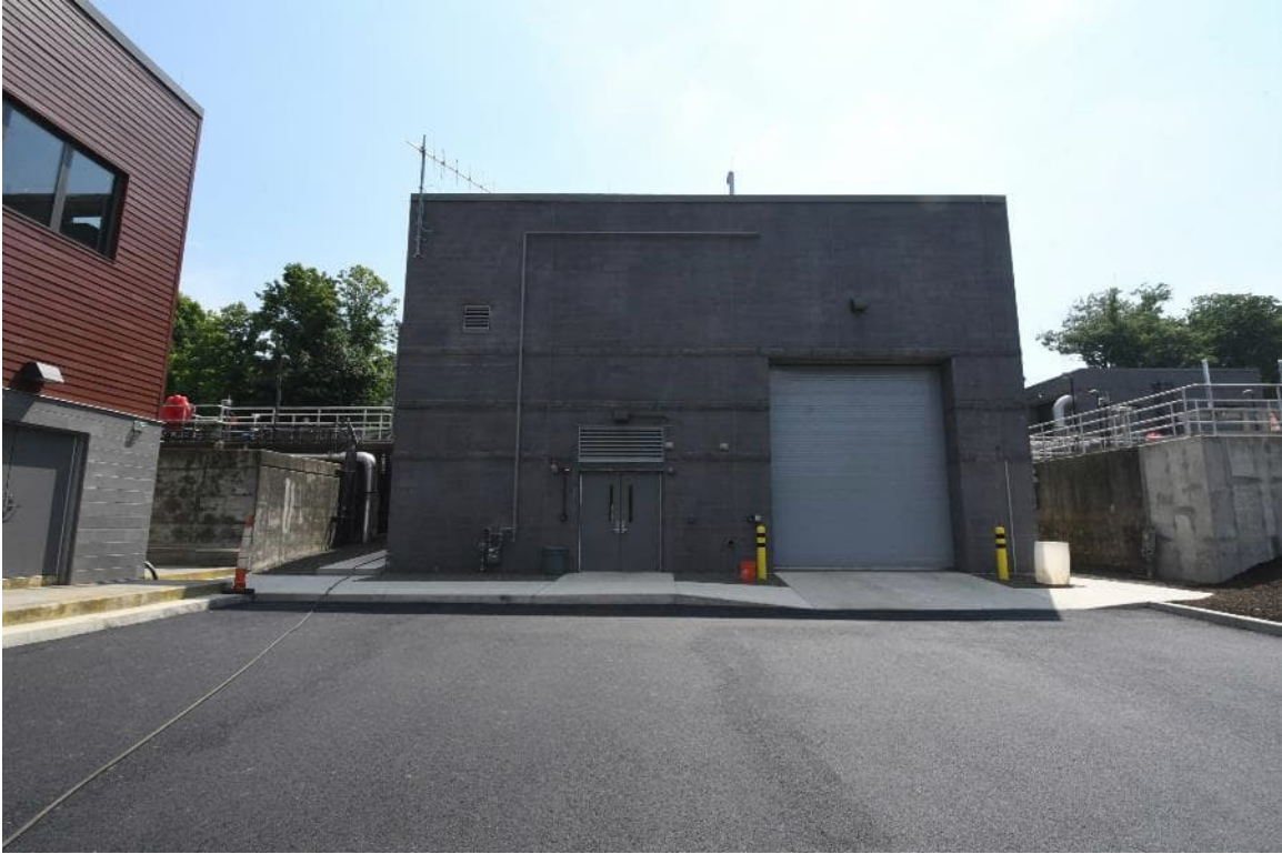
Blower Building and Maintenance Garage
