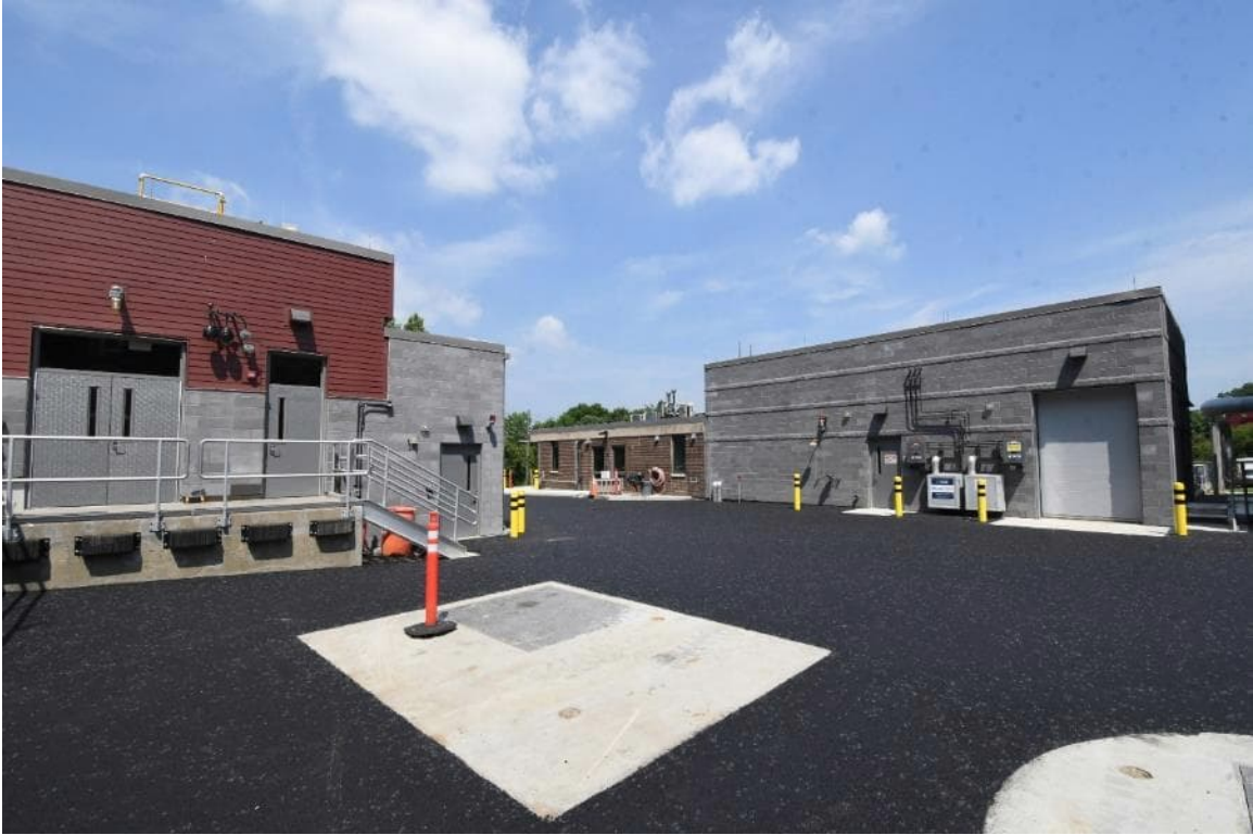
Influent Building (left) and Chemical Control Building (right)
